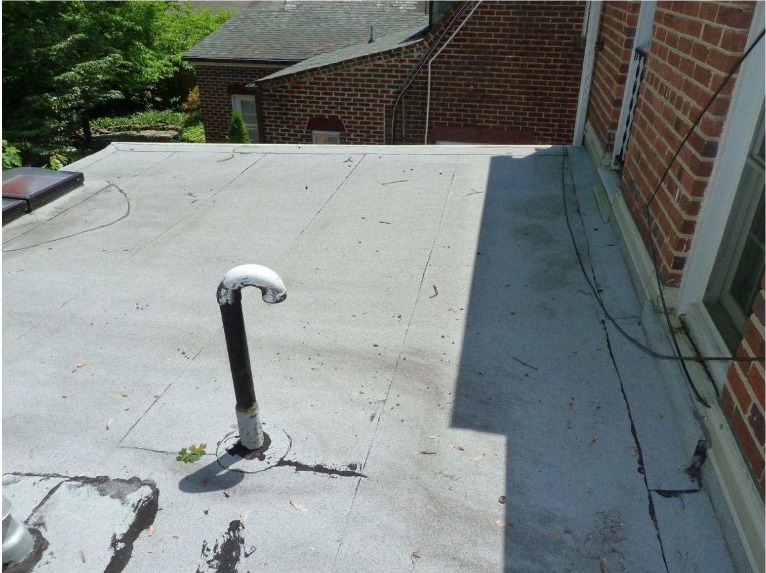
Before Roof over Kitchen
