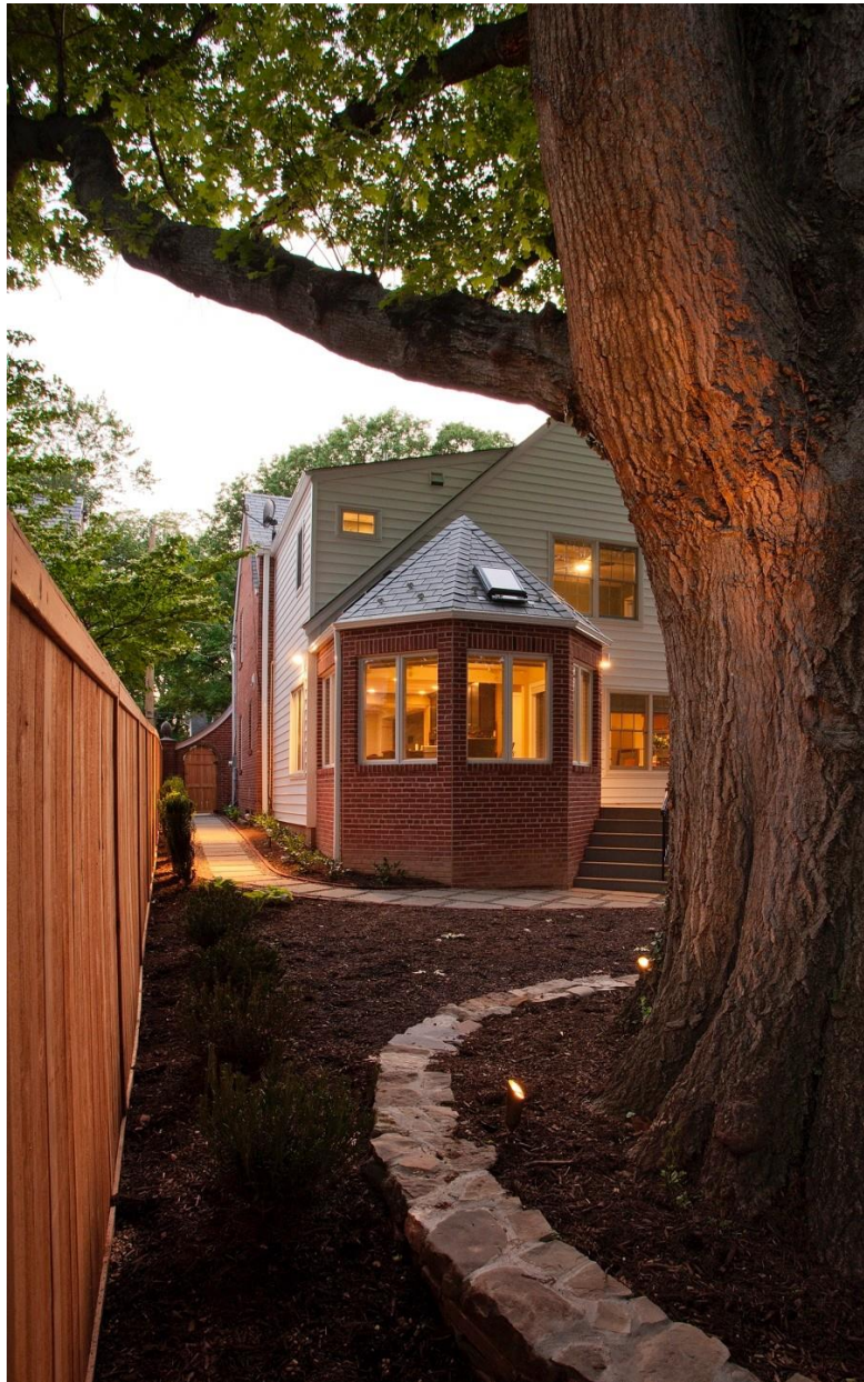
After Rear Elevation from Left
